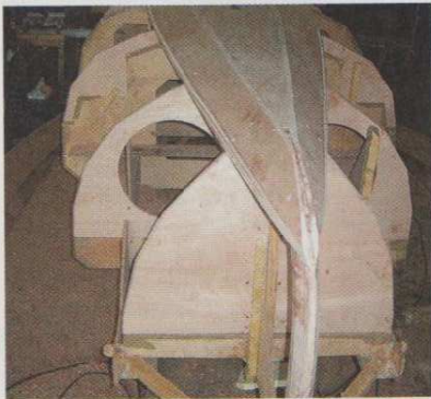
7 The first strake is attached. Planks come in two parts with pre-cut finger scarfs which are glued together before fitting. Note the lower land has been bevelled to receive the next plank.
