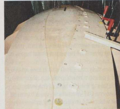
9 Temporary screws with wooden and metal washers hold the strakes in place while the glue is drying. They'll be removed once the glue has cured, and the holes sealed with epoxy.
