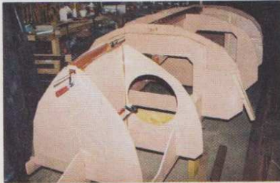
2 The first step is to set up the jig including bulkheads and frames, which slots together and ensures everything is correctly lined up.
