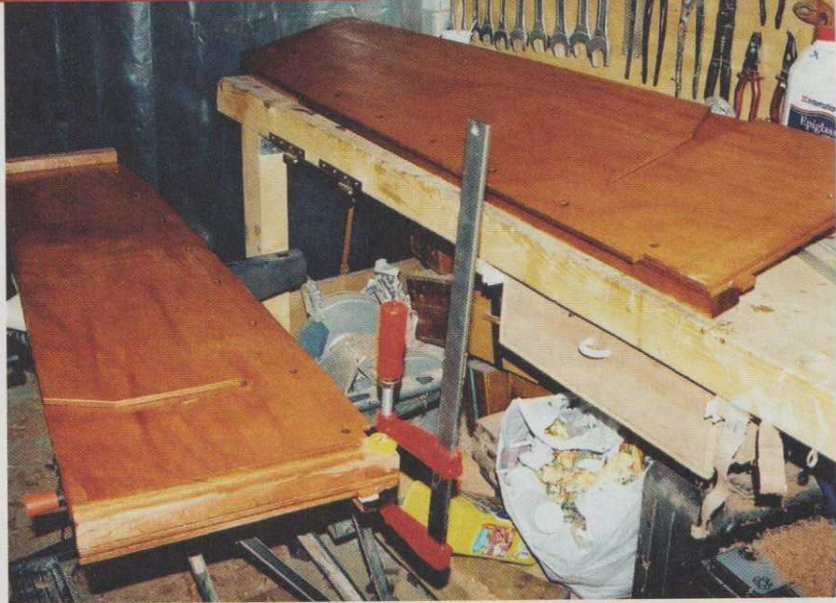
3 The centreboard case is also assembled and fitted at this point. The inside surfaces are sealed with epoxy, as they'll be difficult to access once they're in place. Note the slots for the centreboard pivot.
